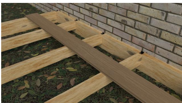
Decking board positioned
