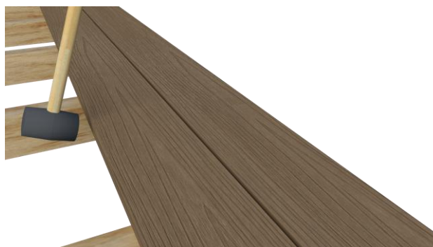
Next board pushed into position
