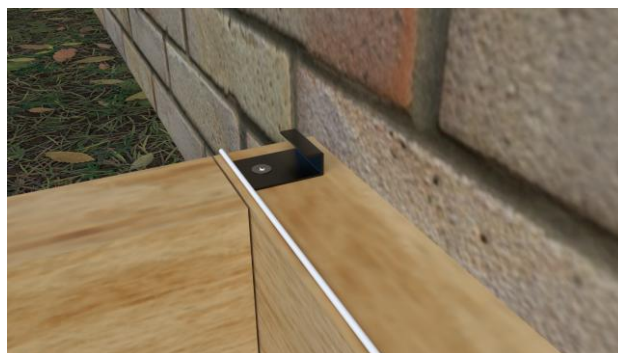
Align and mark the Start/Stop Clip positions across all joists
