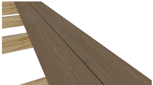
Next board pushed into position
