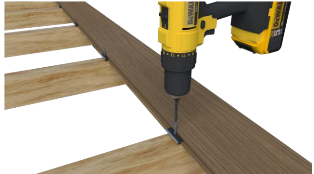
ProLock clip in the groove, screwed down 2 mm
