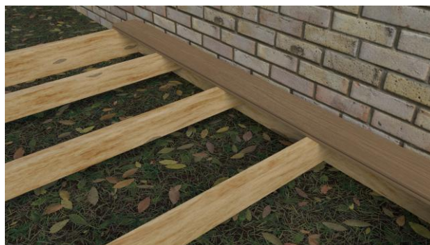
Decking board pushed securely into position.
