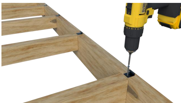
Start/Stop Clips fixed and aligned on every joist along the leading edge
