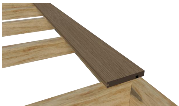
Lower the Edge board carefully, ensuring the clips sit inside the bottom groove of the board.
