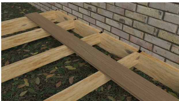
Decking board positioned
